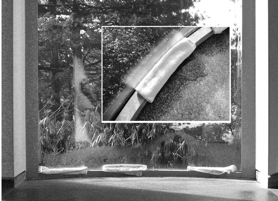
**Figure 10** Museum window in a cold climate (climate zone 6). The prudent humidity limit to avoid condensation depends on airtightness and the R-values of all the components, including window frames. In this building, the 50°F (10°C) DPT was too high to avoid persistent condensation. (*Courtesy Mason-Grant Consulting*)
