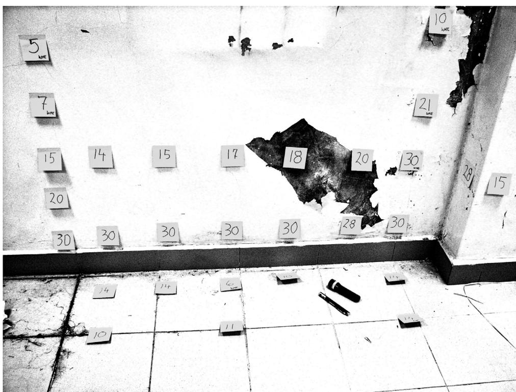
**Figure 8** A moisture map provides visual documentation of locations and the extent of excessive moisture. Using a capacitance-based moisture meter, sticky notes, and a marker, an investigator can document the extent and locations of excessive moisture in a display of “moisture geography” that helps managers locate and eliminate a problem at its source.
